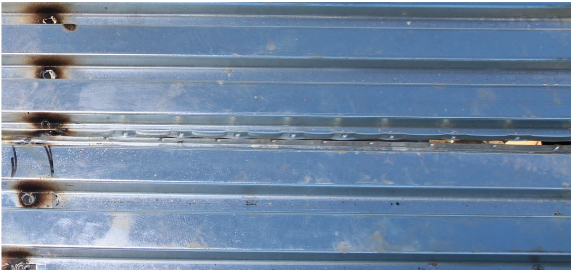
(c) Middle Portion of South Side Lap Connection
