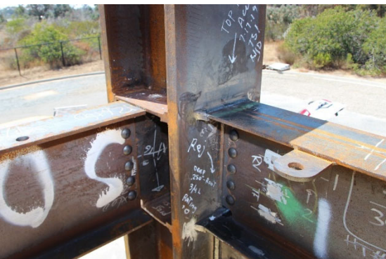
(g) Field Bolting and Field Welding
