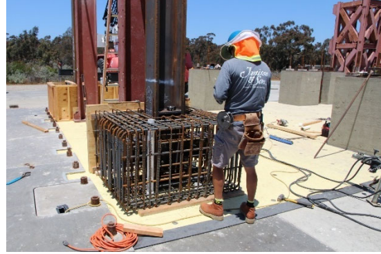
(b) Steel Cages and Formworks for Column 1
