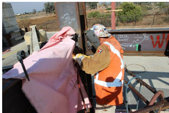
(h) UT Inspection and Welding Repair
