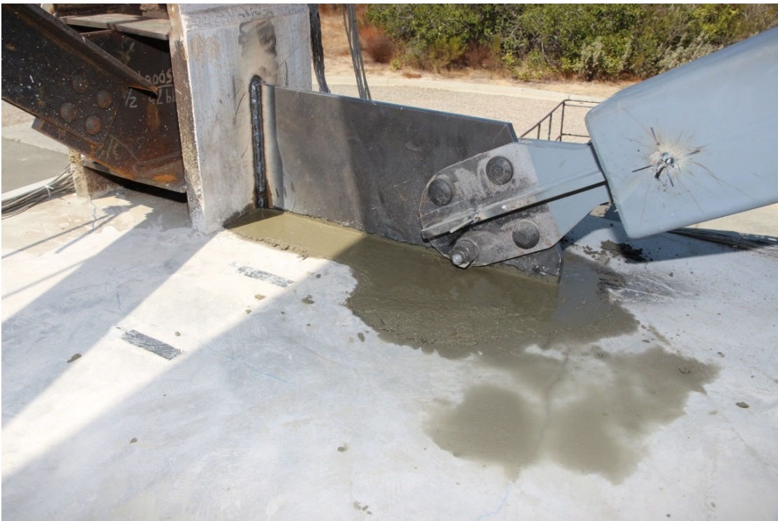
(b) after Grouting
