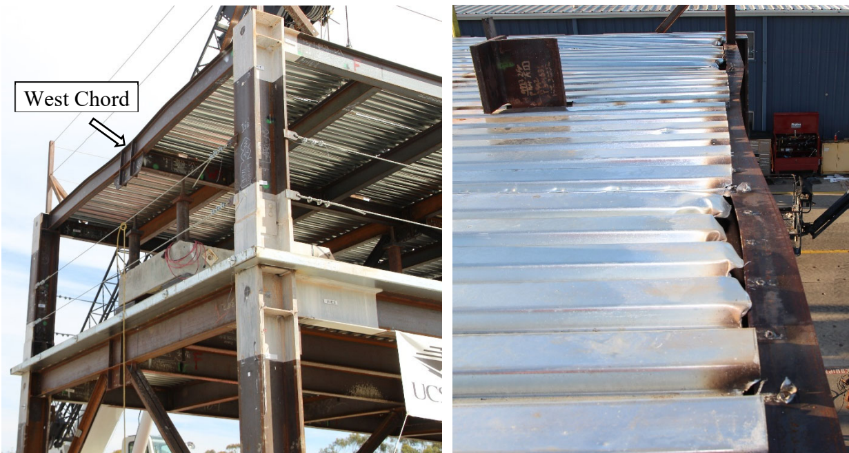
Figure 9.22 Residual Deformation of Roof West Chord
