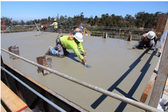
(m) Finishing for Concrete Slab
