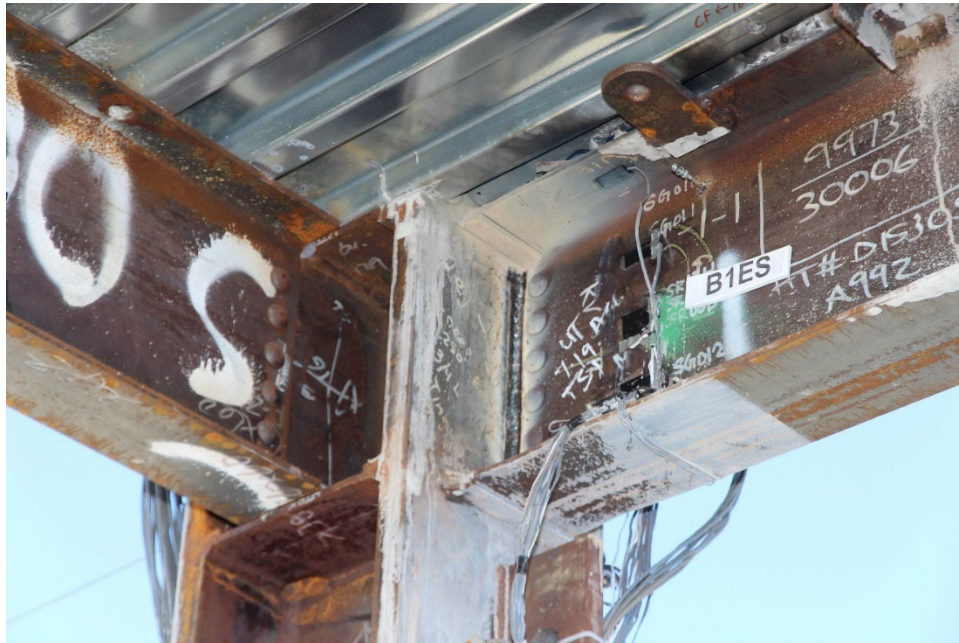
(b) Modified Collector-to-Column Connection
