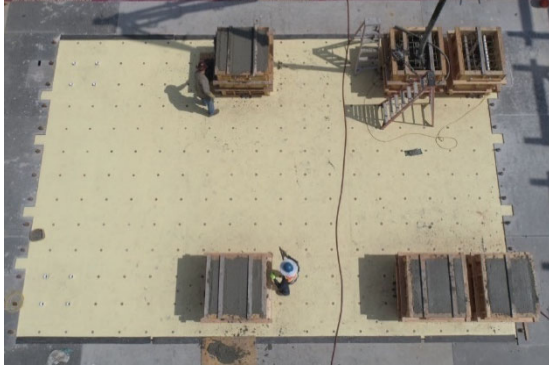
(a) Construction of RC Footings 2 and 3
