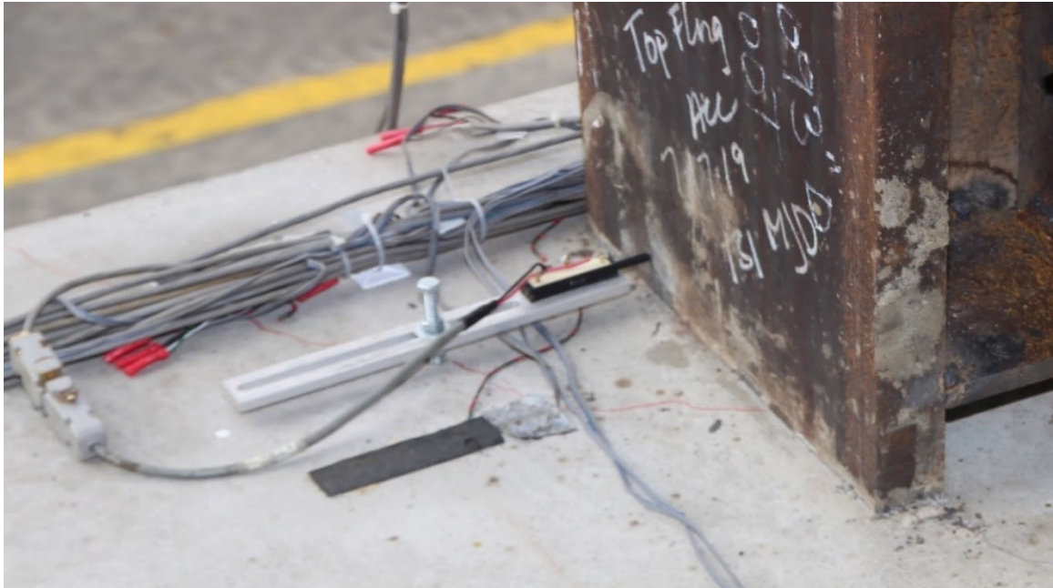
Figure 3.38 Displacement Transducer Installed between Slab and Column
