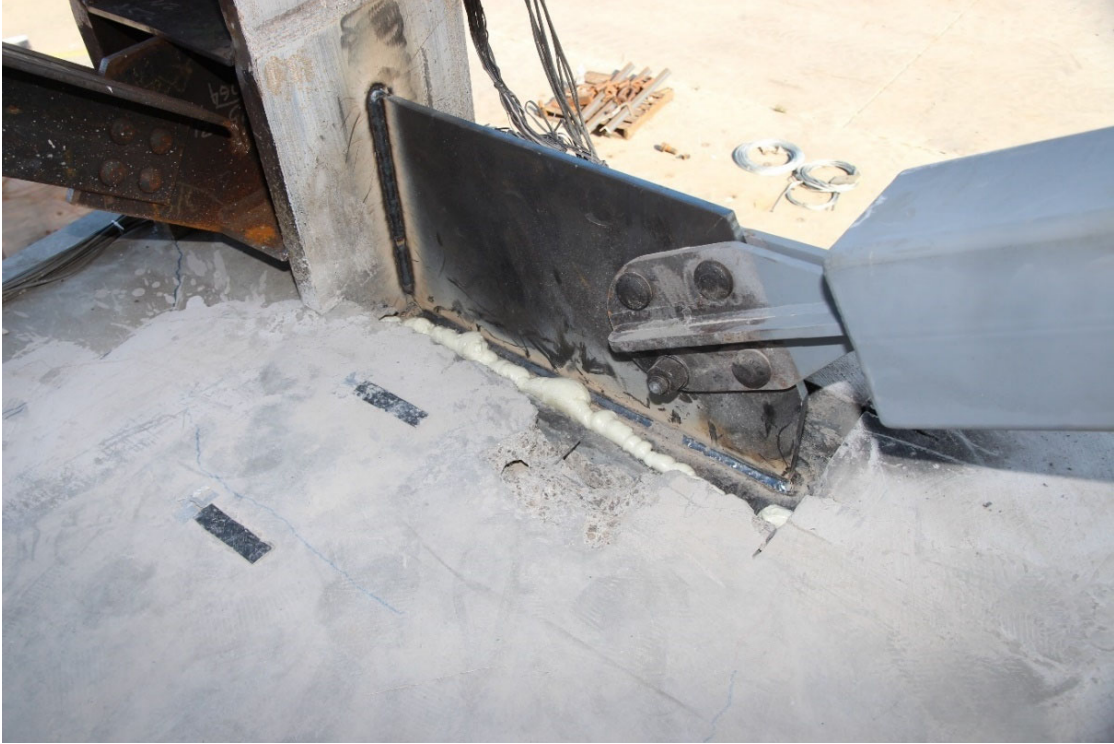
(a) before Grouting
