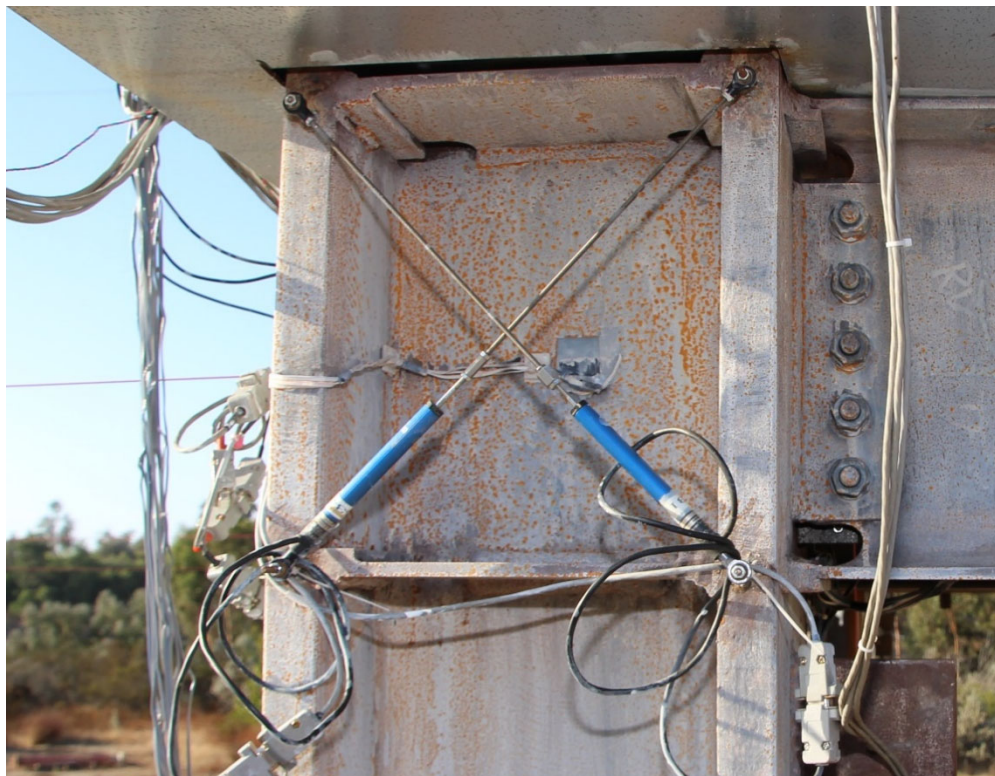
Figure 3.41 Displacement Transducers Installed at Cantilever Column Panel Zone
