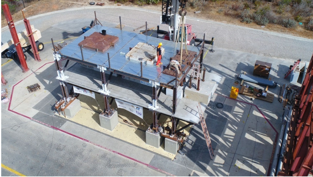
Figure 6.13 Placement of Added Mass Steel Plates
