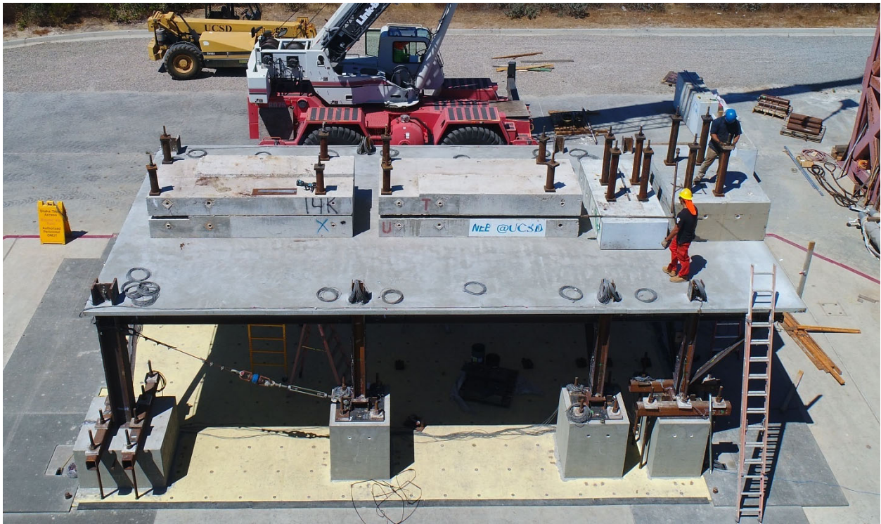
Figure 3.19 Photos of Phase 1 Test Setup
