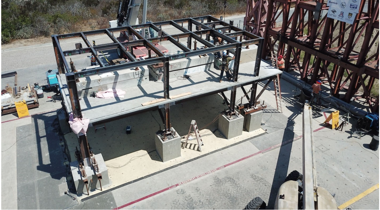
Figure 6.8 Erection of Second Story Frames
