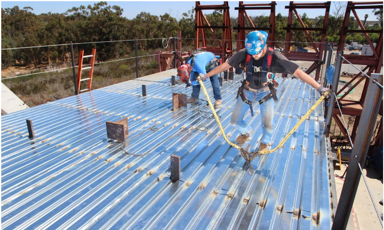
Figure 6.9 Installation of Roof Metal Deck
