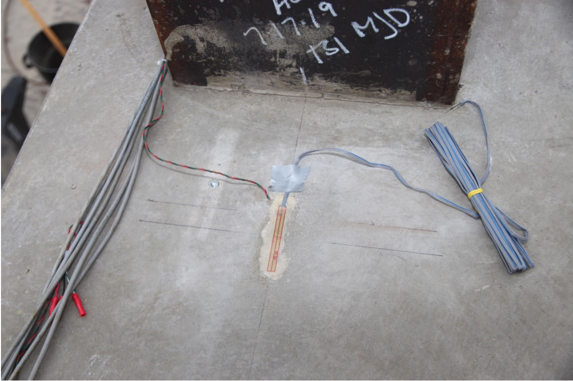
Figure 3.36 Concrete Surface Strain Gauge
