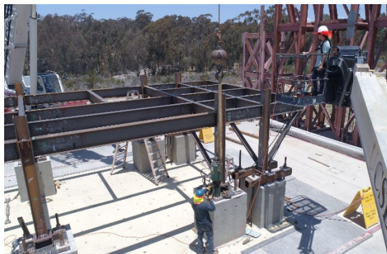
(f) Tensioning of Post-tensioning Rods
