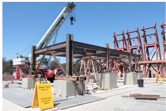
(e) Erection of Steel Frame
