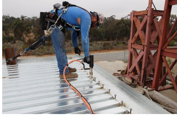
(j) Welding of Headed Anchor Stud
