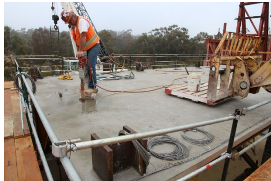
(n) Core Drilling of Concrete Slab
