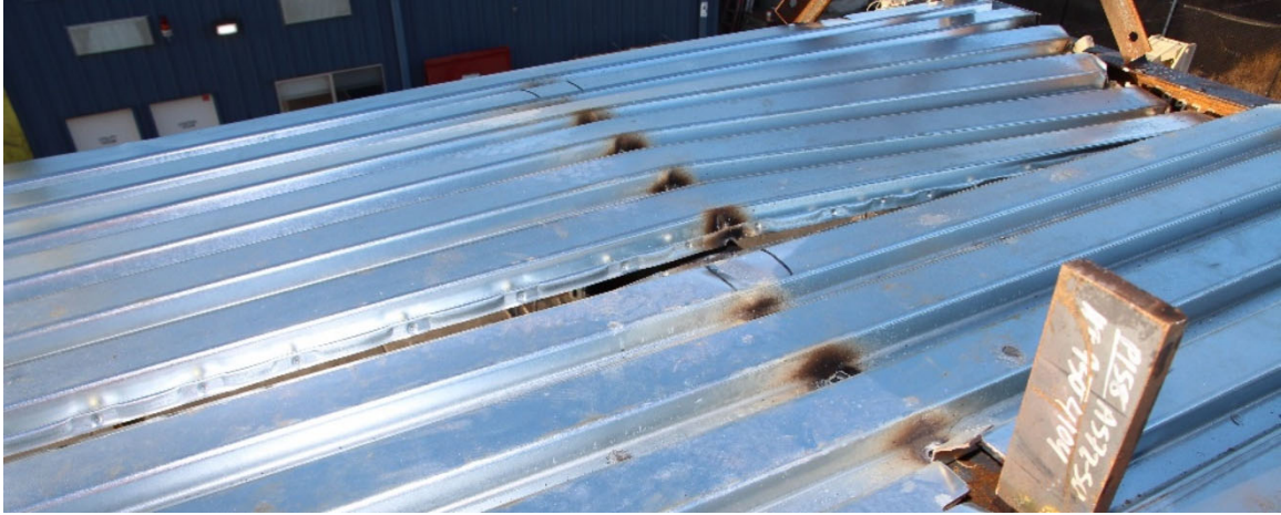
(a) near Southwest Corner
