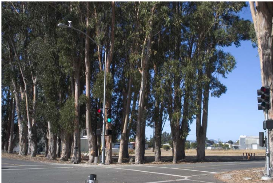
Figure 8.10 Traficon Video Camera at PATH RFS Intelligent Intersection
