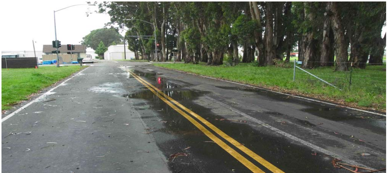
Figure 8.12 PATH Testbed with Standing Water
