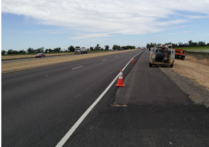
Figure A.10: PH04 on-site location photograph.
