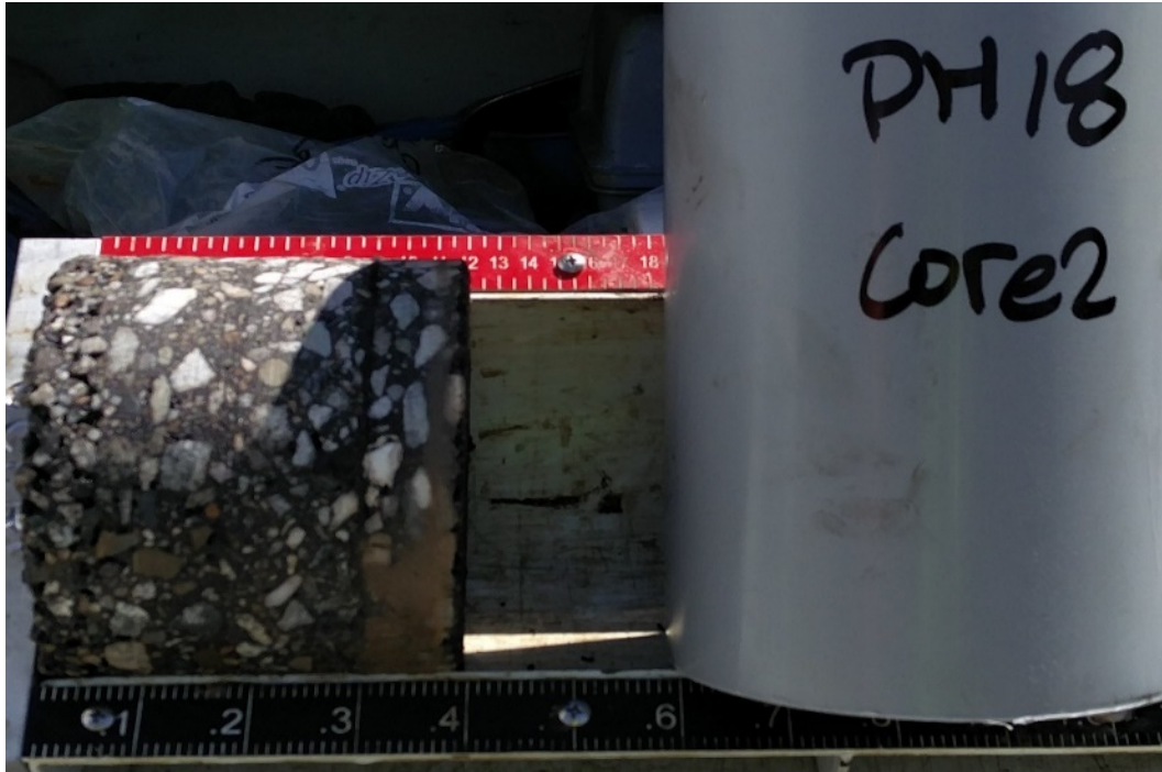
Figure B.31: Pavement core sample for PH18.
