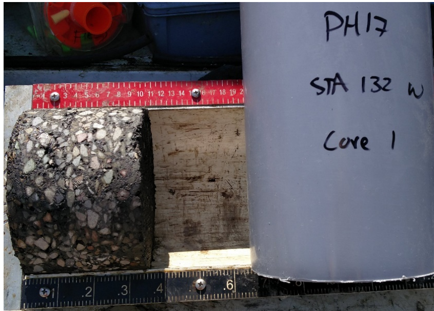
Figure B.28: Pavement core sample for PH17.
