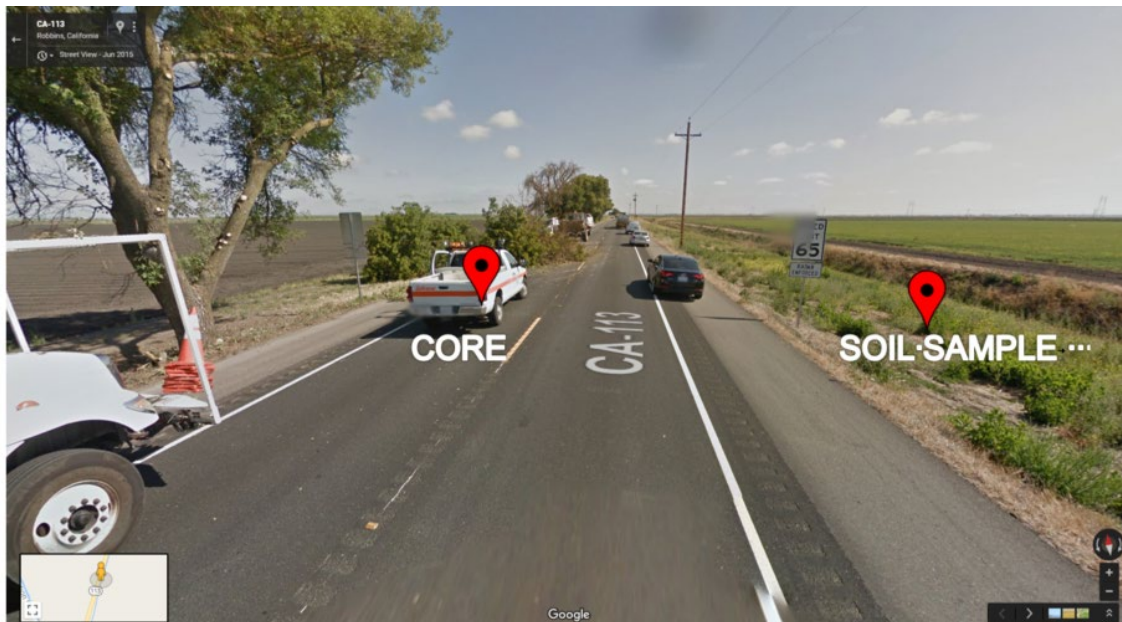
Figure B.12: Pavement core and subgrade soil sample locations for PH10 from Google Maps.
