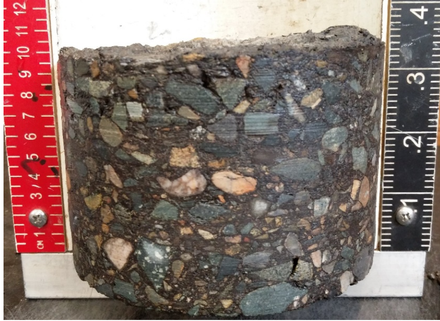
Figure B.21: Pavement core sample for PH14.
