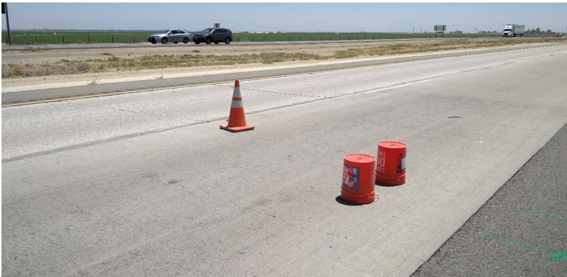
Figure A.41: On-site location photograph of PH20 (right lane) during Caltrans closure.
