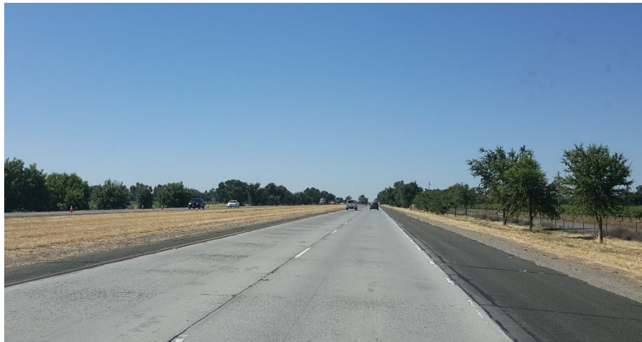
Figure A.5: On-site location photograph of PH02.
