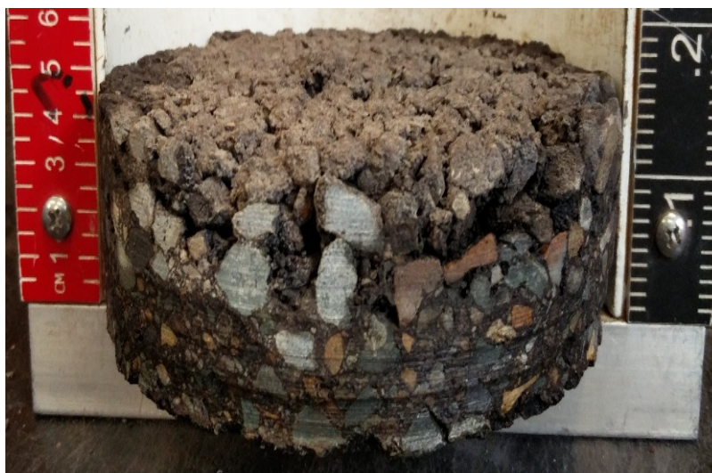
Figure B.19: Pavement core sample for PH13.
