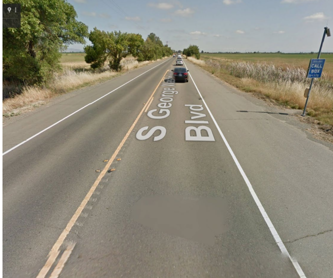
Figure A.24: On-site location photograph of PH11 (right lane) and PH12 (left lane) from Google Maps.
