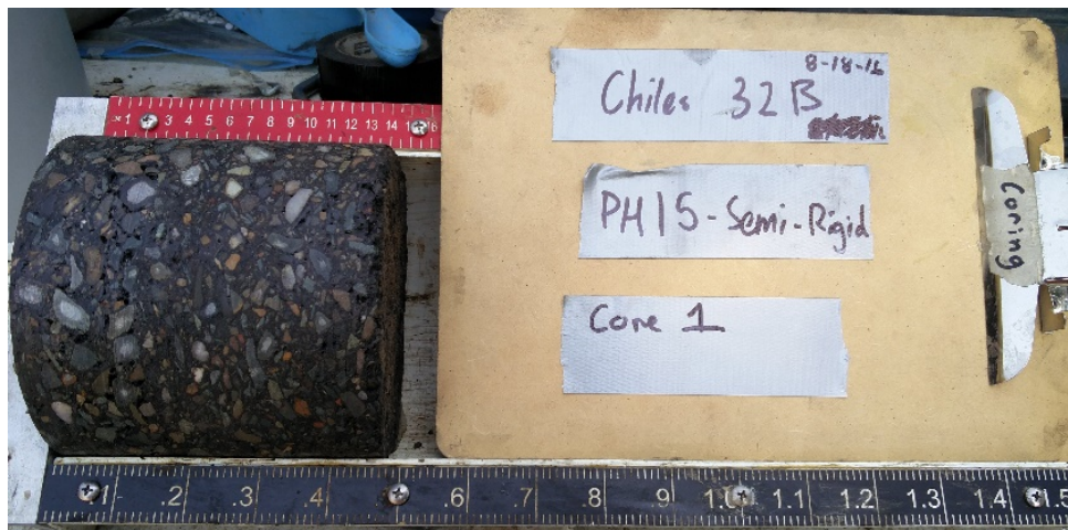
Figure B.23: Pavement core sample for PH15.
