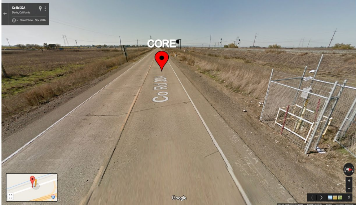
Figure B.37: Pavement core sample location for PH23 from Google Maps.
