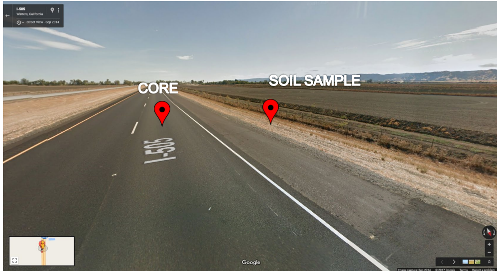
Figure B.5: Pavement core and subgrade soil sample locations for PH04 from Google Maps.
