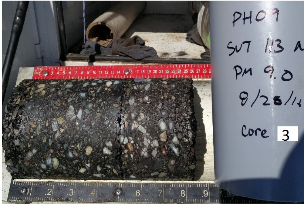
Figure B.11: Pavement core sample for PH09.
