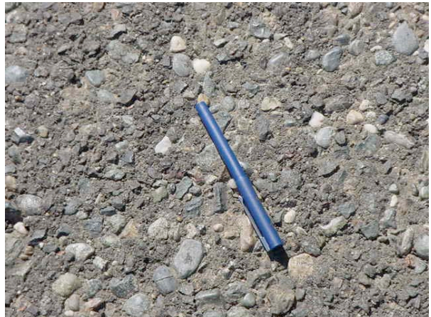
d. Asphalt pavement surface, magnet location prior to coring
