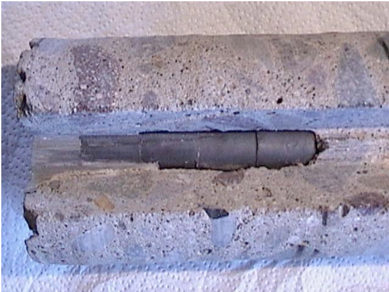
Figure 3.1: A cut through a plug installed in a PCC pavement.
