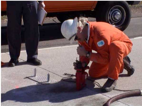
c. Core extraction, concrete pavement
