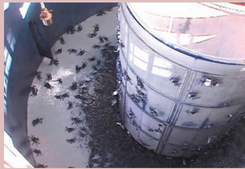
This fish salvage tank is supposed to hold fish diverted from the Bay-Delta. Instead, it is clogged with mitten crabs.
