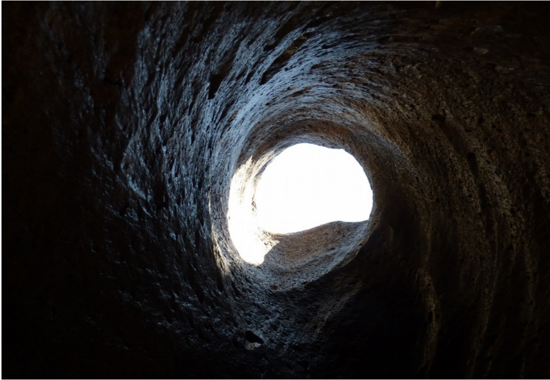
Figure6. 49: Swirling eroding patterns inside void with Panel 2, looking upward.
