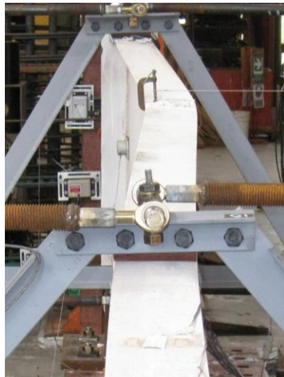
Figure 5.21 CS2 Initial Buckling of Inner Flange (+3.5 in., 1 st Cycle)
