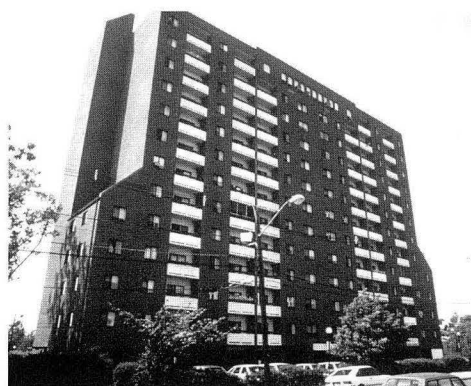
Figure 1. The Margolis Apartments in Chelsea, Massachusetts, was designed in 1973 and is typical of high-rise construction from that period. This USHUD project is the site of ventilation and infiltration measurements to improve comfort and energy performance.
