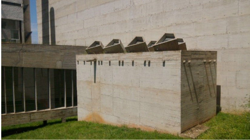
Figure 5.2 A view from south-east of the seven “machine guns” protruding from the roof of the sacristy. Four in the front row, and three behind. (Photo by author in May 2016).
