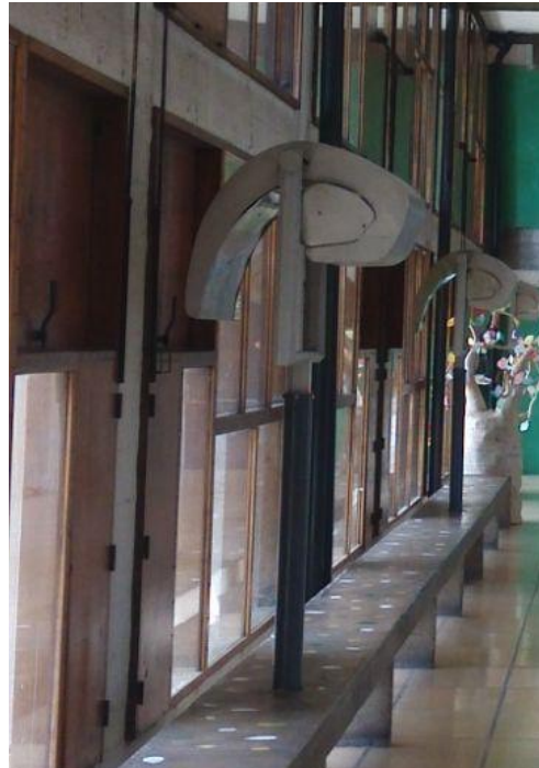
Figure 5.10 Large snail-shaped lighting fixture (1951-52) along the corridors of the Unité d'Habitation Marseille (photo by author in May 2016)
