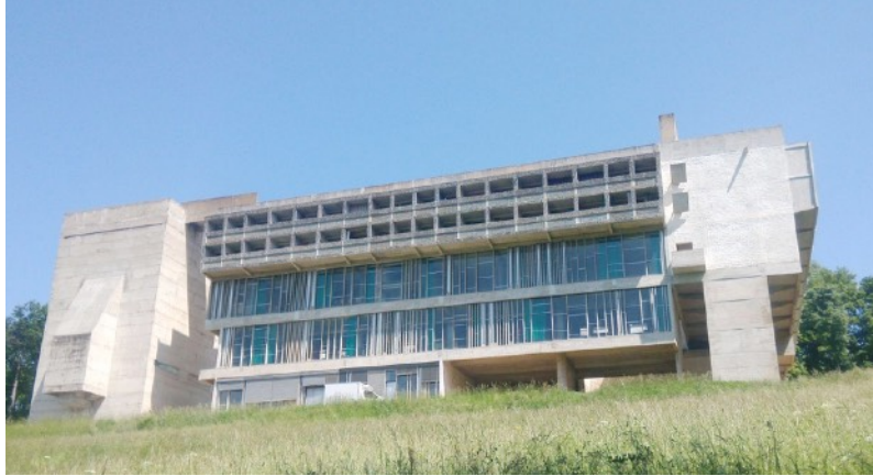
Figure 5.9 A view of the west façade. Two levels of modular house unite on the (Photo by author in May 2016).
