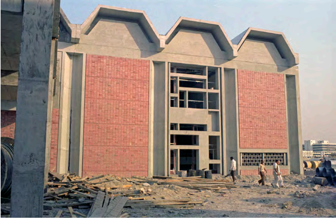
Figure 23: A photograph of Kuwait National Museum showing the redbrick cladding and one of the window patterns. Source: Aga Khan Award for Architecture.
