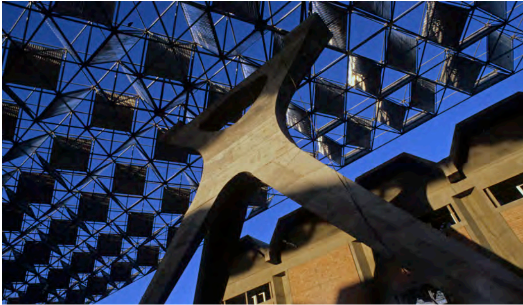
Figure 19: A close-up photograph of one of the columns with the four legs (a symbolic form of a camel) of the Kuwait National Museum showing. Source: Aga Khan Award for Architecture.
