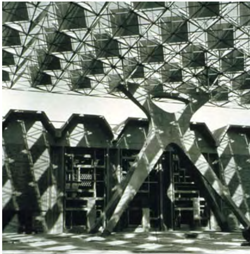
Figure 127: Photograph of Kuwait National Museum's space-frame and tensile shadings demonstrating the play of shade, shadow, and light on the museum's buildings and one of the columns (the columns meant to represent a camel figure). Source: Aga Khan Award for Architecture.
