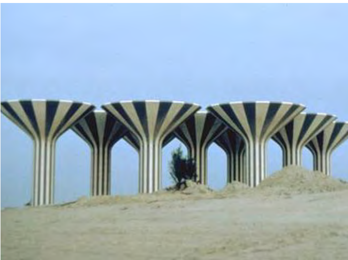
Figure 92: Photograph of Kuwait Water Towers. Source: Aga Khan Award for Architecture.
