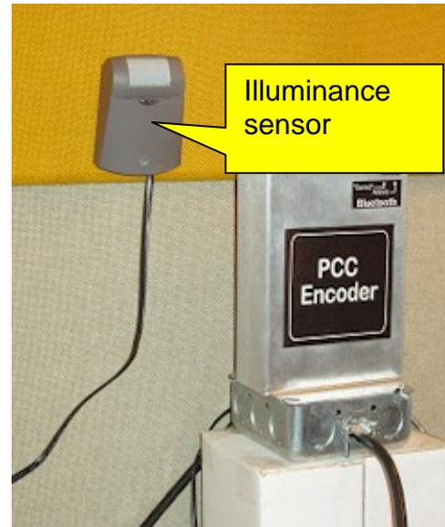
Figure 6. Closer view of the PCC Encoder and attached junction box (which collectively form the "intelligent junction box"). Also shown to the left is the environmental sensor that is attached to the wall. Note the location of the illuminance sensor within the environmental sensor.
