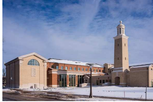
Figure 17 John Simpson, Walsh Family Hall at the University of Notre Dame, 2018, Indiana, United States
