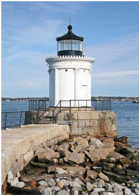
Figure 13 Thomas U. Walker, Portland Breakwater Lighthouse "Bug Light," 1855, Maine, United States
