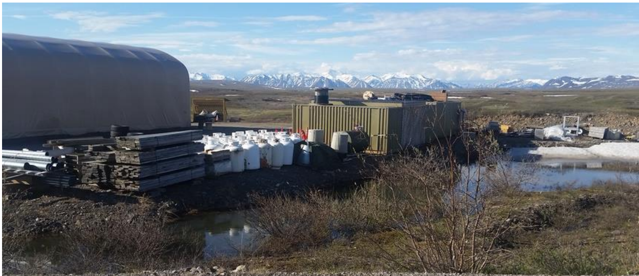
Figure 22 Cold Storage is surrounded by building materials and other items from past or for future use.
