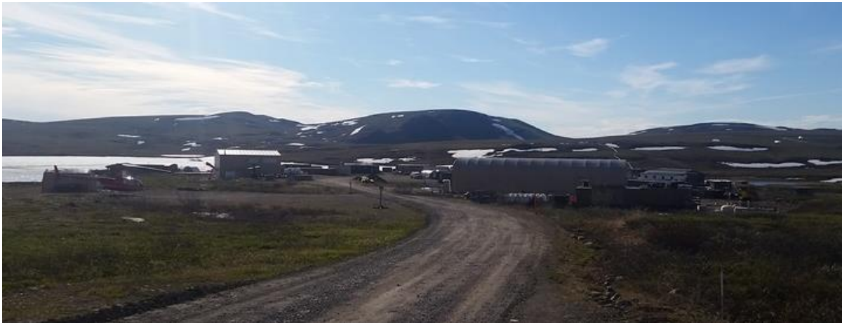
Figure 31 The utilitarian nature of the station is immediately evident on entering PRS.
