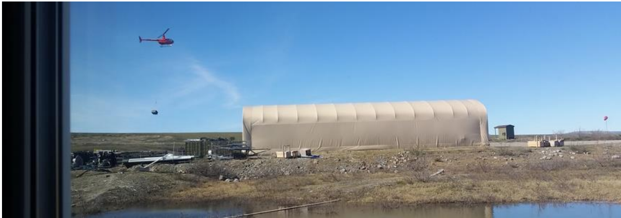
Figure 21 Helicopter moving materials near Cold Storage.
