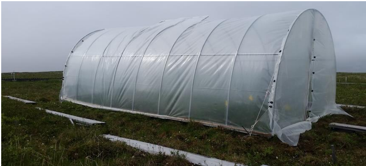
Figure 44 The same greenhouse from Figure 40 after we completed repairs.
