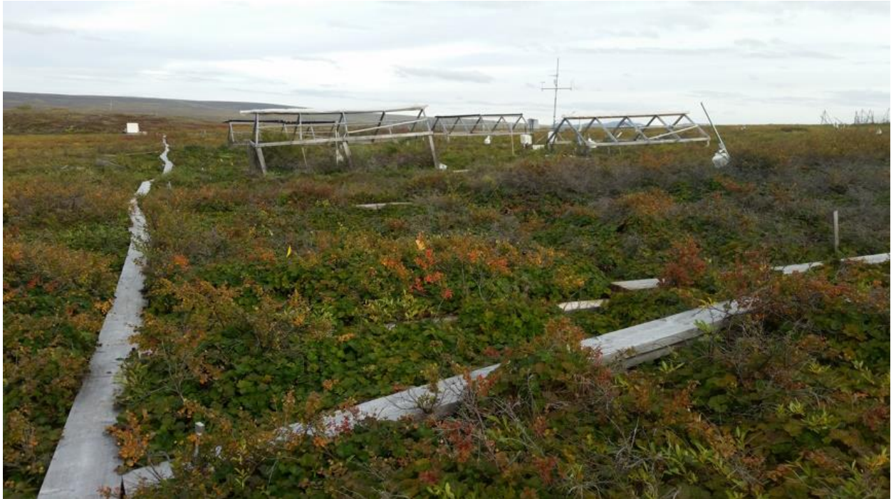
Figure 41 The tundra overtaking greenhouses and shadehouses that have been warped by the harsh Arctic weather.
