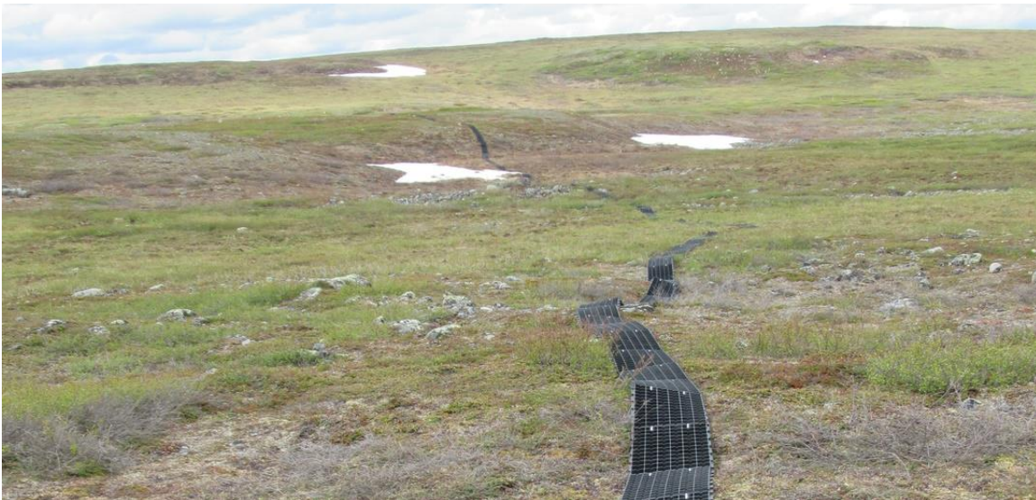
Figure 36 A Geoblock path stretching away into the tundra.
