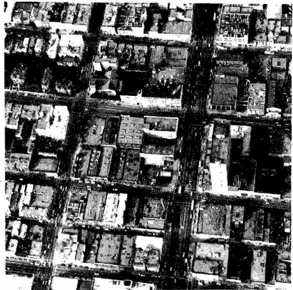
Aerial Photo of the Van Ness Avenue Area
