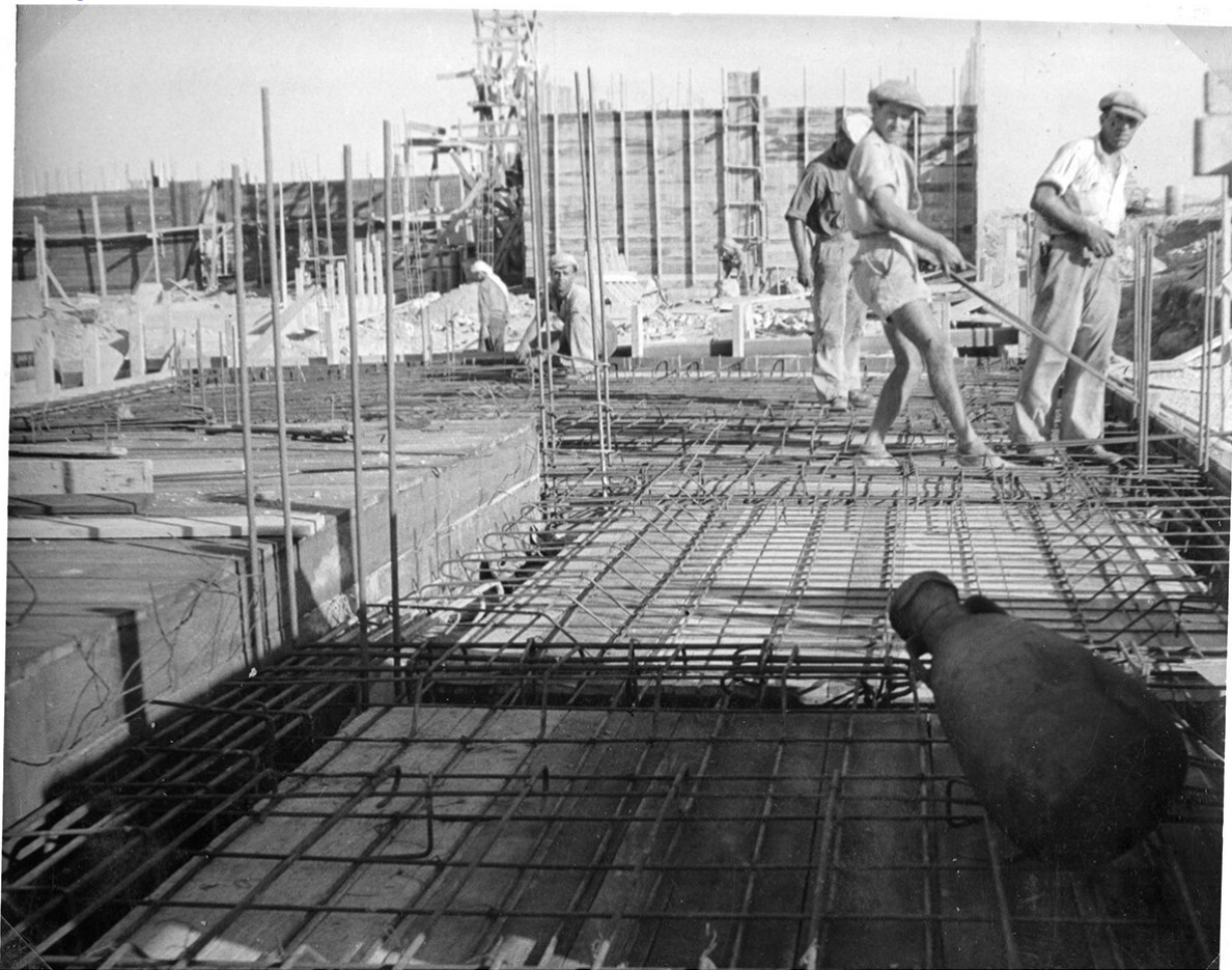
Fig. 10. The Lajjun Tegart Fort under construction in June 1940; Israel State Archive, file 58585
