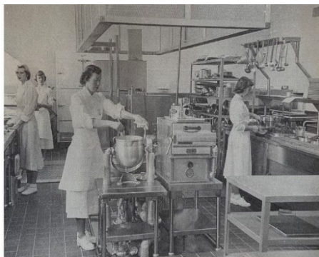
4 Nutrition lab in the new Home Economics Building, 1954
