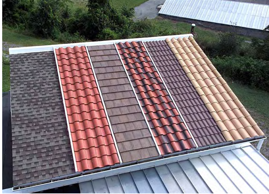
Fig. 2. An assembly of steep-slope attics was placed on top of the ESRA and clay and concrete tile were installed by the Tile Roofing Institute.
