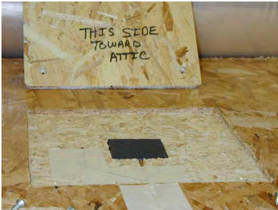
Fig. 6. Heat flux transducer embedded in the roof deck for measuring the heat flow penetrating through the roof tile and into the attic.
