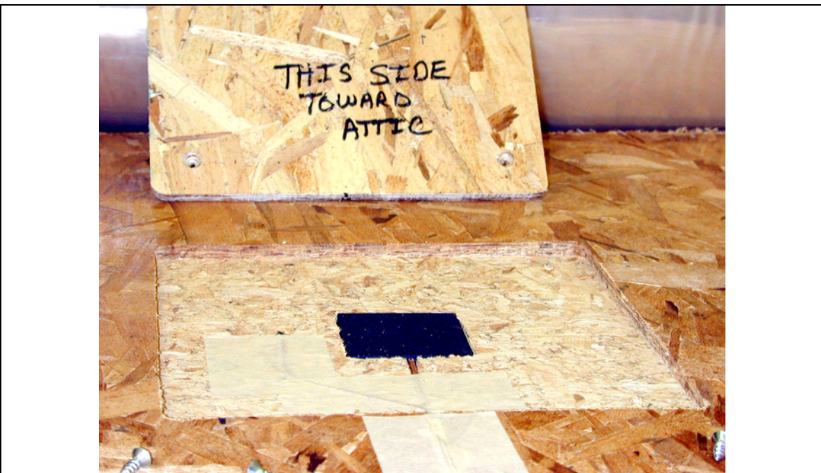
Figure 6. Heat flux transducer embedded in an OSB guard and used to measure heat flow crossing the roof decks of the demonstration homes.
