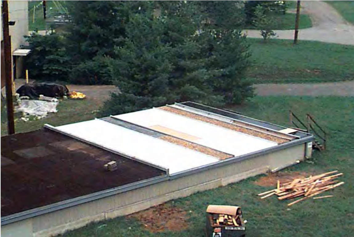
Fig. 1. Envelope Systems Research Apparatus (ESRA) is a one-story building for testing low- and steep-slope roof products.
