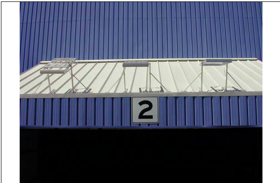
Figure A.5. Exposure rack mounted on the roof of the Steelscape warehouse in Richmond, CA.
