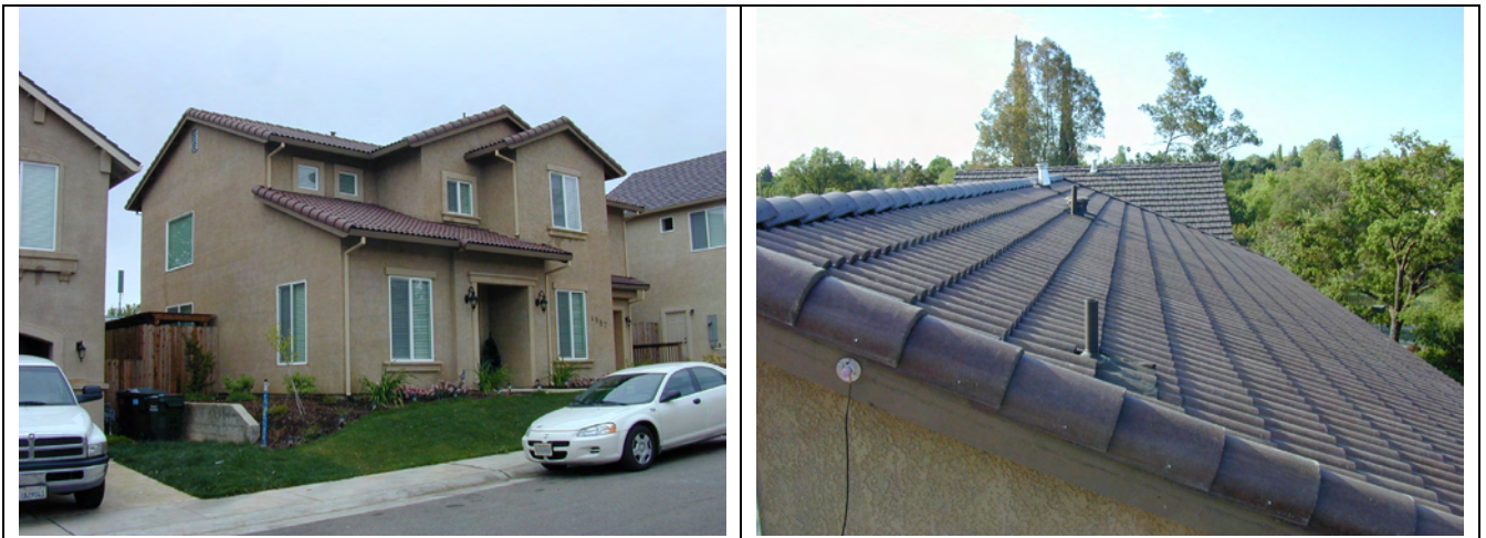
Figure 4. Finished A-style home demonstrating Hanson Hacienda concrete tile after retrofit painting by American Rooftile Coatings.
