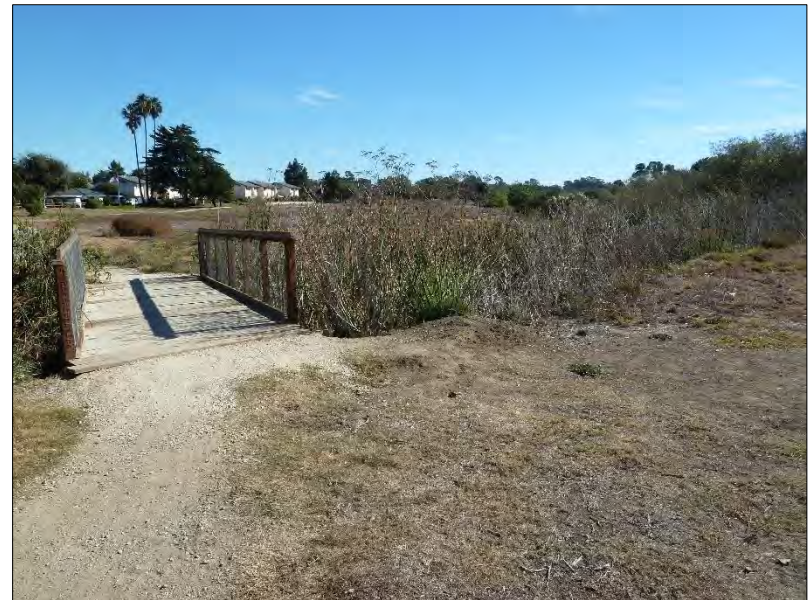
Photo 16: View east at Phelps Creek bridge crossing and confined channel. 9/30/2015
