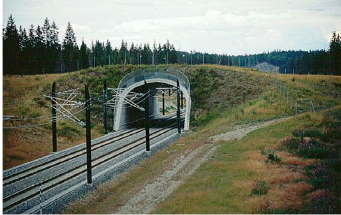
Fig. 3. Overpass in Norway over train. (Photo by B. Iuell)
