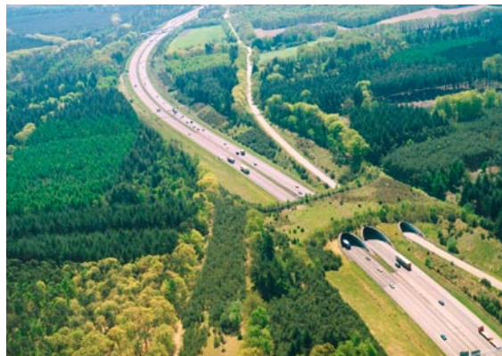
Fig. 1. Transportation infrastructure can fragment habitats, but building fauna passages can mitigate habitat fragmentation. (Photo by Peeters and Slagboom BV)
