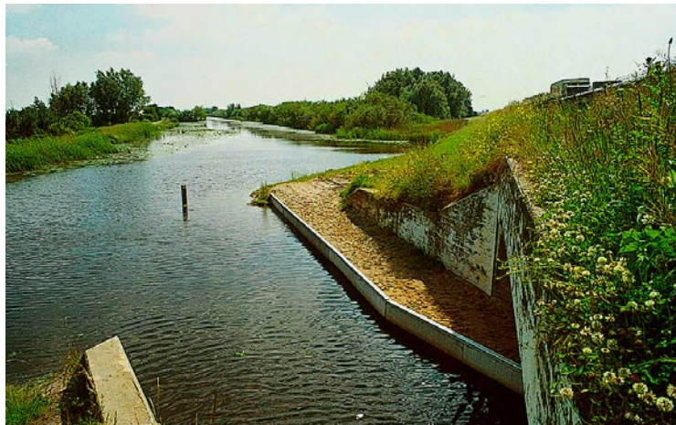
Fig. 2. Adapted bridge under highway in The Netherlands. (Photo by H. Bekker)
