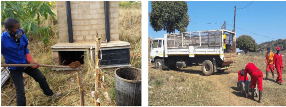
FIG. 2. Emptying and transporting of UDT sludge (Mercer and Buckley, 2019). UDT, urine-diversion toilet.
