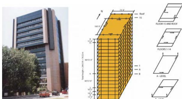
Figure 1: The Factor building and its seismic array. Arrows show locations and polarities of sensors on each floor.
