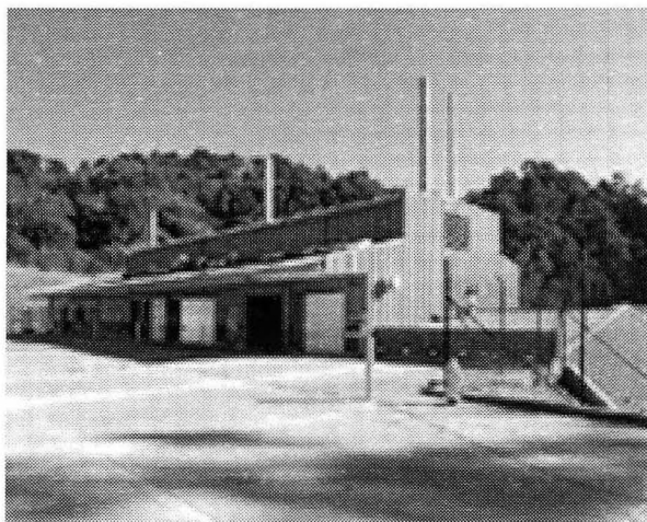
Upper yard at the new Hazardous Waste Handling Facility.
