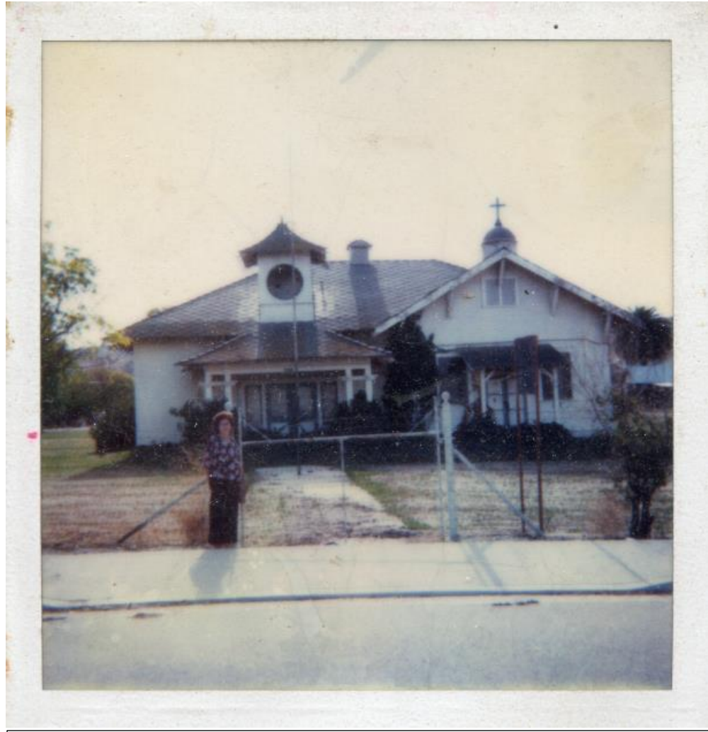
Figure 34: Rey standing in front of the Bryn Mawr School building, ca 1960. By this time the school had been turned into a church and then left empty until the 2000s. (Courtesy of the Loma Linda Area Parks and Historical Society, Coyazo Collection)
