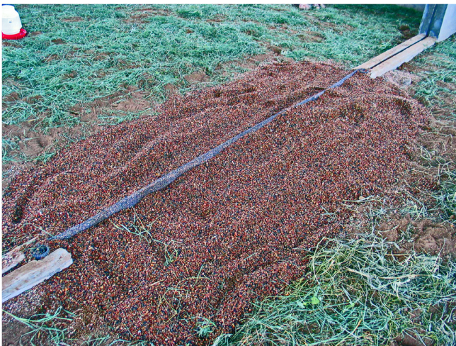
B. Pea gravel-filled trench below ground.
