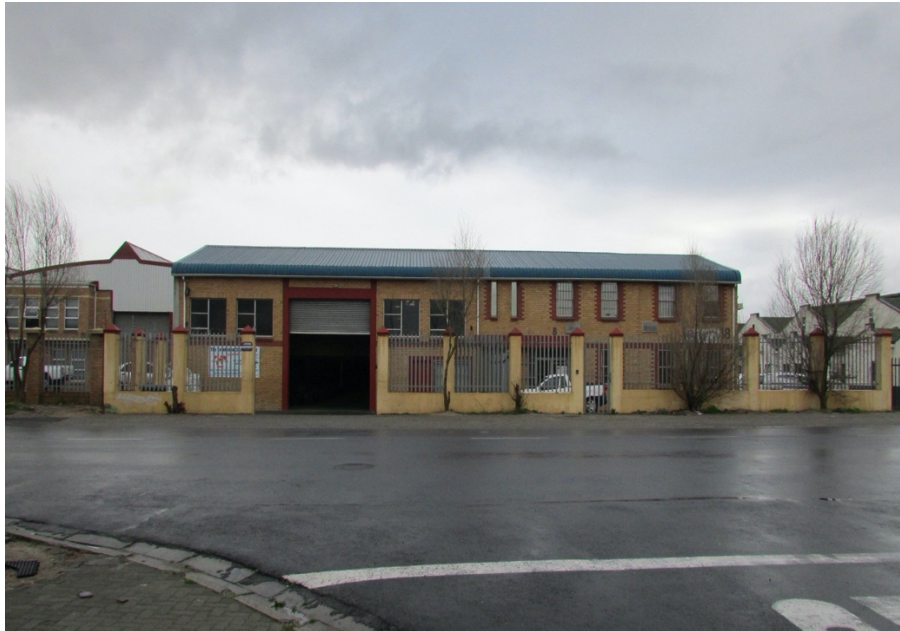
Figure 6: Previous RRO Building in Airport Industria, Cape Town (Photo: Author 2017)
