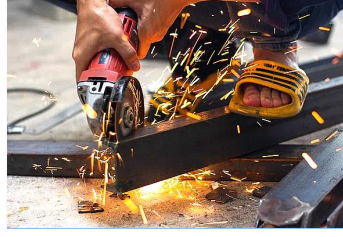
BLIP: A worker is cutting metal with sparks flying. LaDiC: A worker is grinding steel with an angle grinder. Ours: A worker cutting steel with an angle grinder without protective gear.
