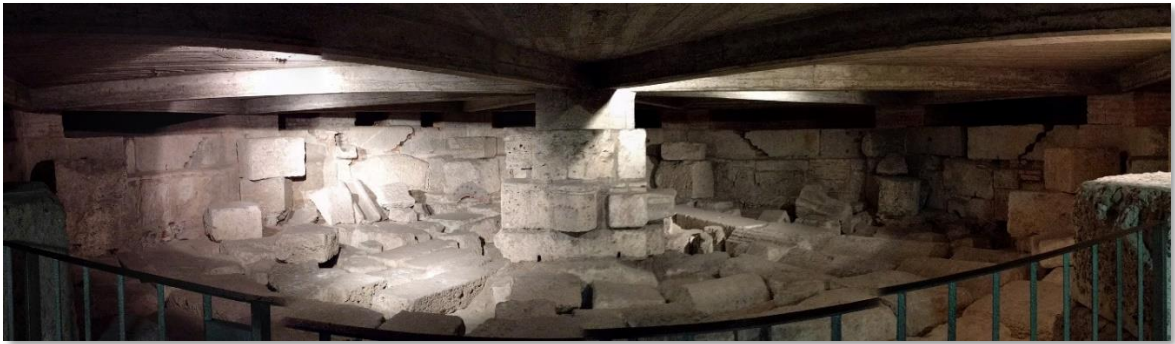
Figure 14. Foundations of South Chapel in the Laurentian complex
