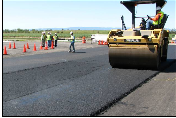
Figure 2.38: Cecabase: Breakdown rolling.
