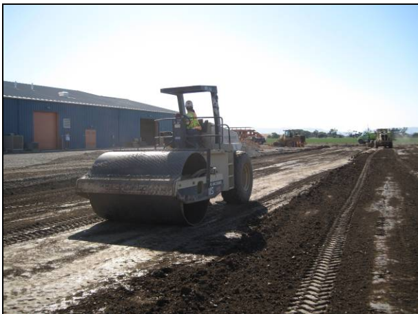
Figure 2.12: Final compaction.
