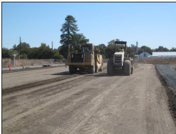
Figure 2.19: Heavy watering prior to pre-final compaction.
