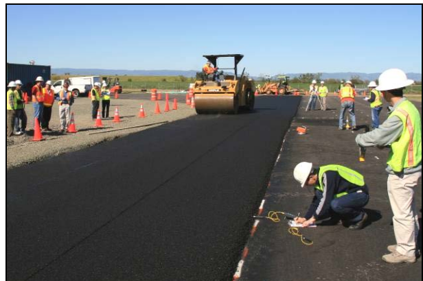
Figure 2.33: Gencor: Breakdown rolling.
