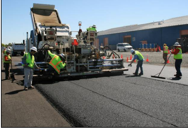
Figure 2.37: Cecabase: No smoke from truck and paver.
