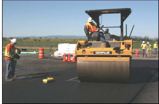
Figure 2.31: Control: Final rolling.
