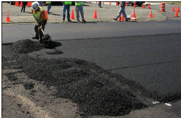
Figure 2.37: Cecabase: No smoke from truck and paver.
