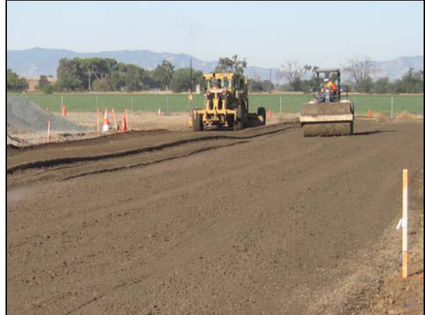
Figure 2.18: Initial compaction.
