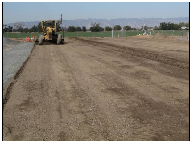
Figure 2.18: Initial compaction.
