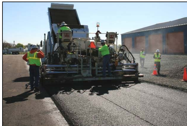
Figure 2.32: Gencor: Smoke from truck and paver.
