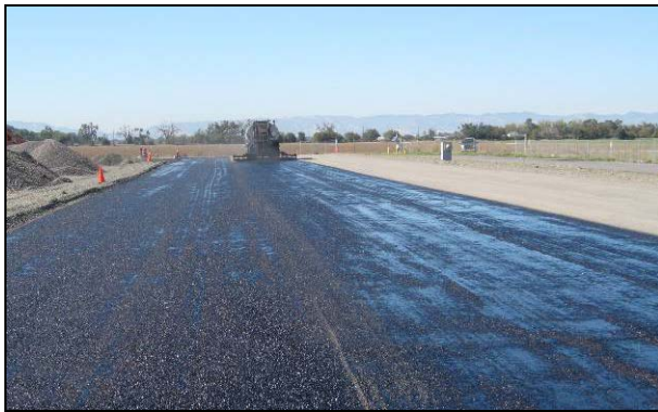
Figure 2.24: Prime coat application.
