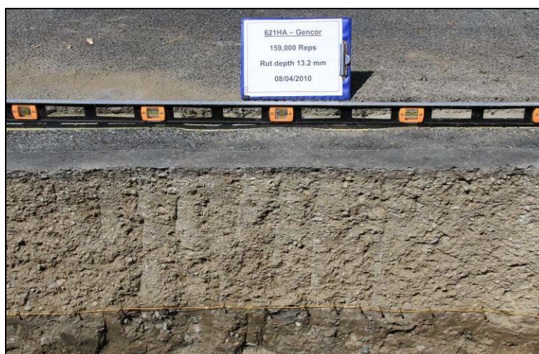
Figure 5.3: 621HA: Test pit photograph.
