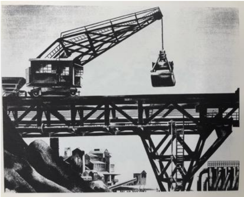
Figure 4. 18 Shimada Yōsuke, Construction Site , 1933 Blue Dragon Society Catalog
