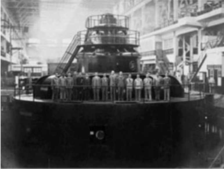
Figure 4. 45 Suihō hydropower turbine, 1940 Toshiba Mirai Kagakukan
