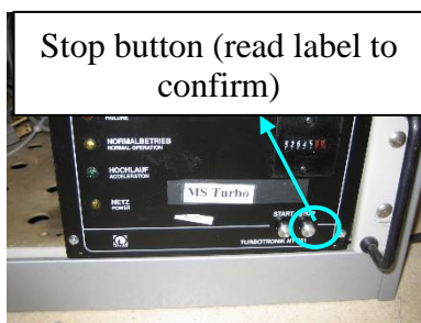
Figure 42. Turbo pump controller emergency shutdown
