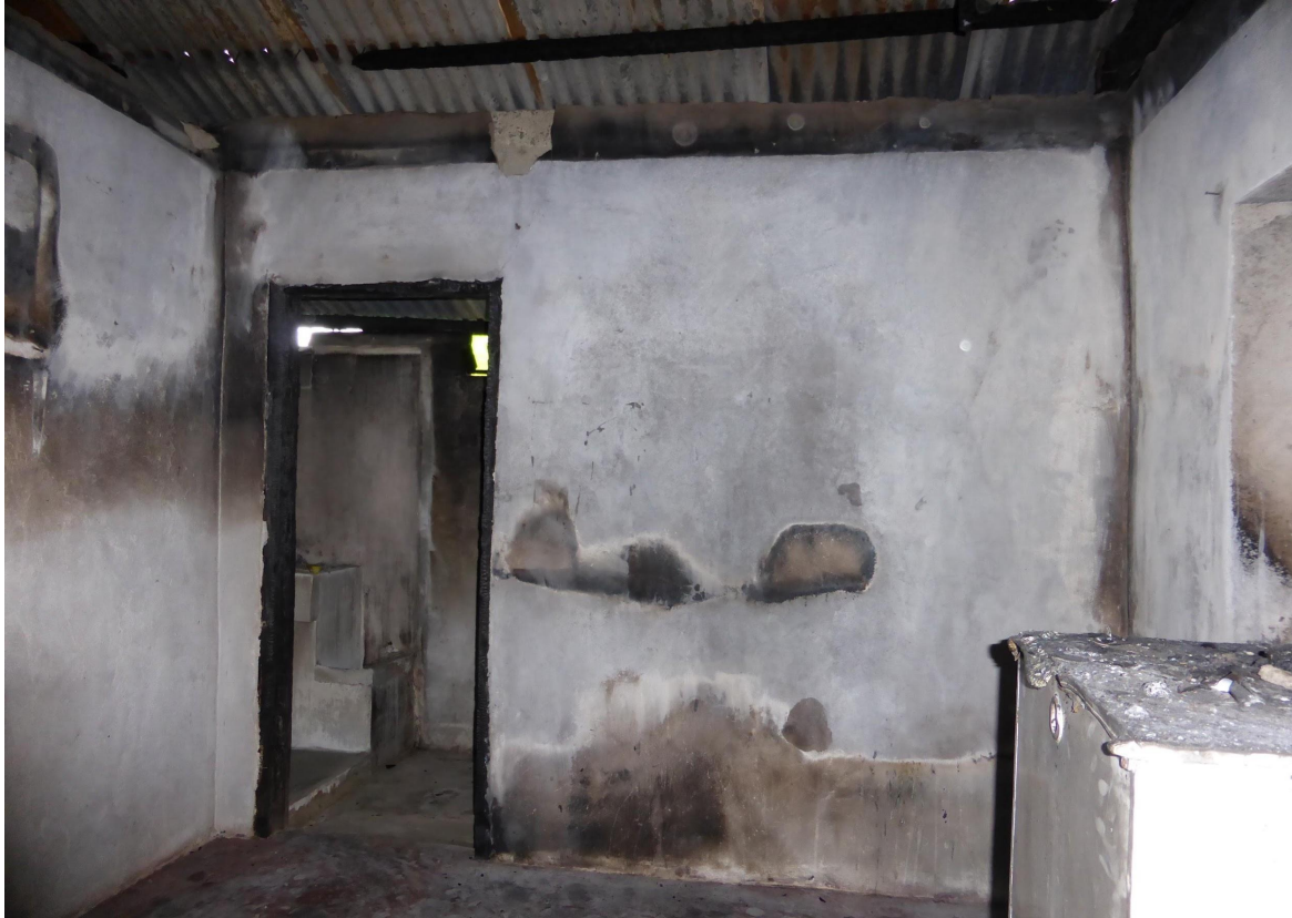
Figure 2.2. This clinic in the Philippines burned down when a candle set the building on fire
