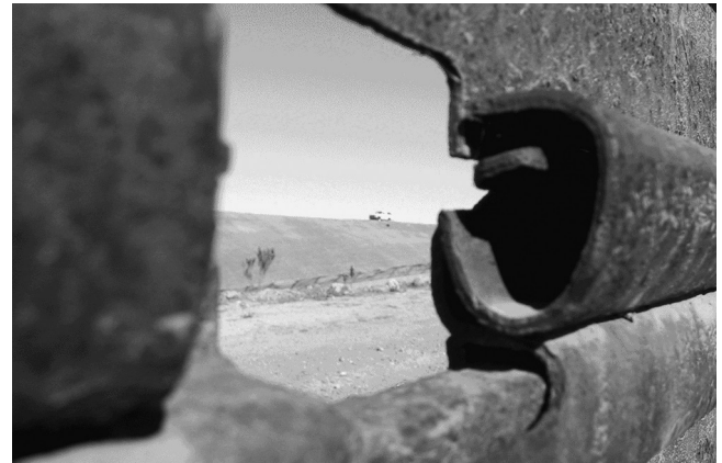
A current section of the US–Mexico border wall built in the 1990s with recycled temporary air-landing mats used in the Desert Storm war in the Middle East. Courtesy of Estudio Teddy Cruz + Forman.
