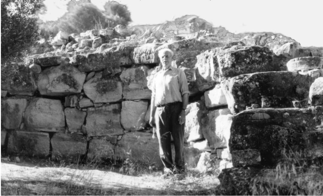
PLATE 8.3. View of cyclopean masonry of Agia Triada Tholos B
