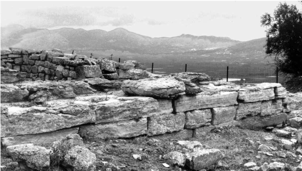
PLATE 12.2. View of gypsum wall blocks on west face of temple on the Gortyn acropolis
