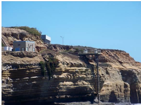
Fig. 6-3. Site seen from the shore
