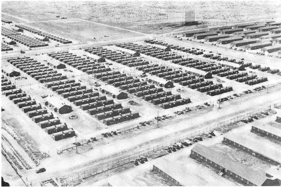
Figure 37. View of Hanford barracks, 1944.
