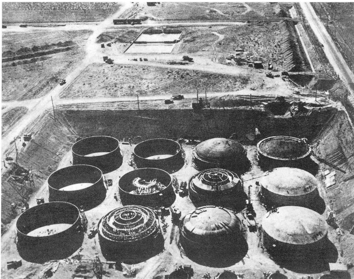
Figure 47. Single shell waste tanks at Hanford, late 1944.
