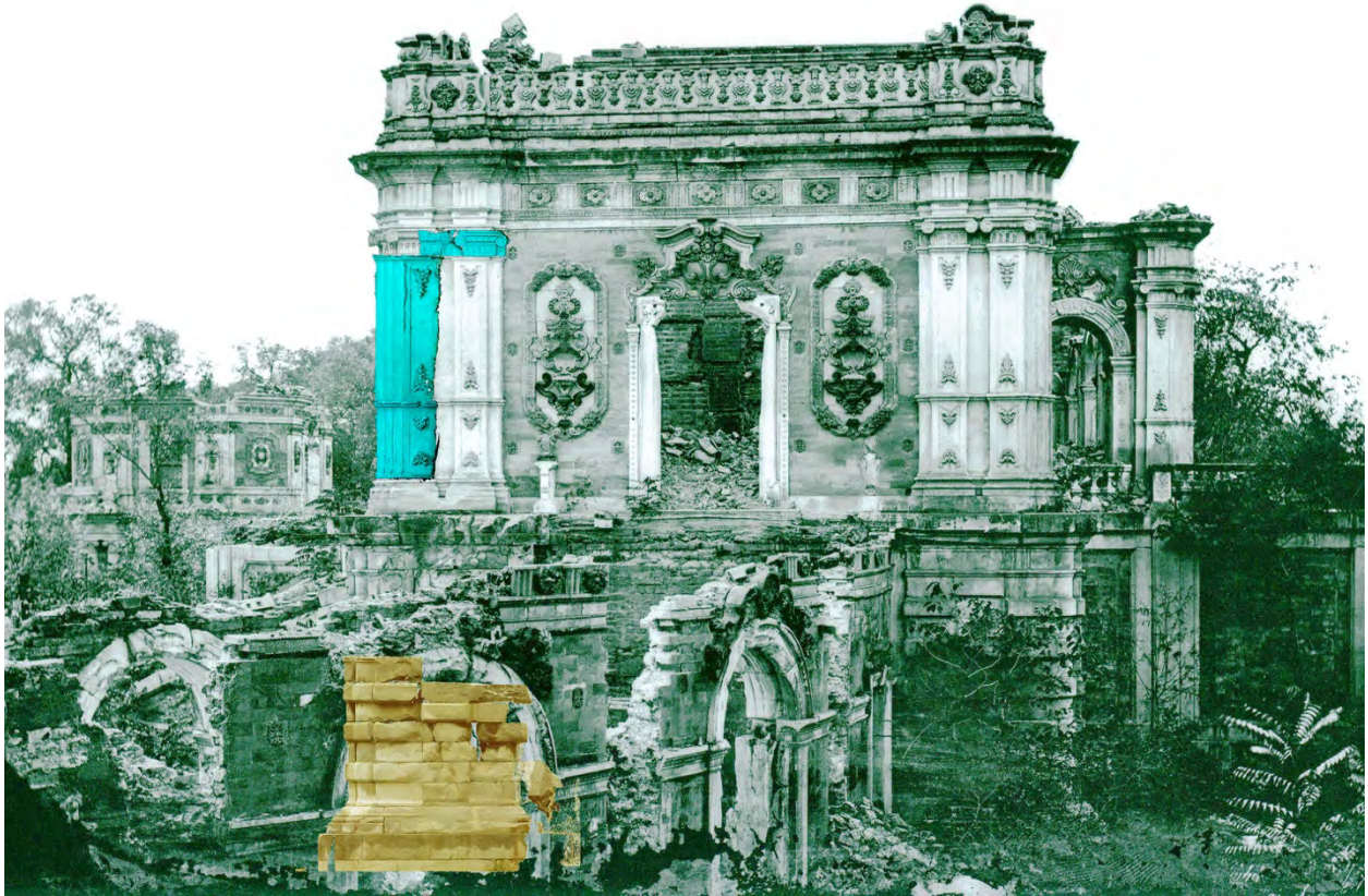
Fig. C.1. Photogrammetric 3D models of fragments from Xieqiqu overlaid on photograph by Ernst Ohlmer.
