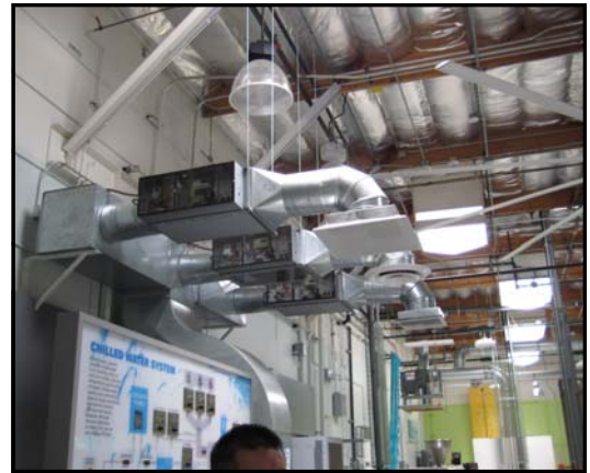
Edison Water Pumping System
