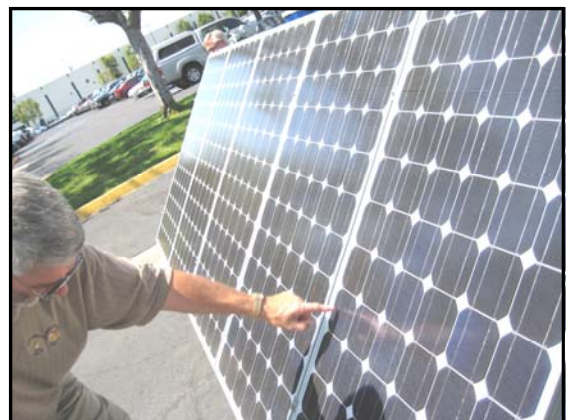
Solar Panels at the IBEW Local 11 Electrical Training Institute
