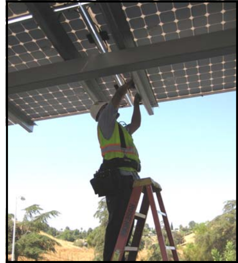
Solar Panel Installation Pierce College
