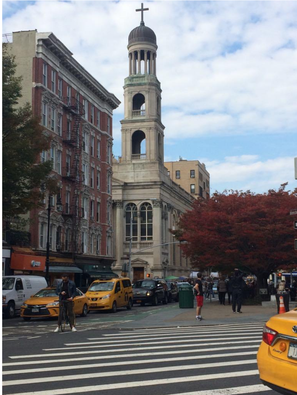
Fig. 7. Our Lady of Pompeii Church, Carmine Street Greenwich Village, September 2015. The church, a safe haven for Italian immigrants, was founded in 1892 and the building constructed in 1928. This perspective of only the three-story bell tower atop the church promotes its stature and dignity, as it stands guard over the lower buildings of the Village. The entire church can be seen from the corner of Carmine and Bleecker, but this perspective can only be seen from the entrance to Minetta Lane Triangle, bordering Bleecker Street and Sixth Avenue. Photo credit: Denice Martone.
