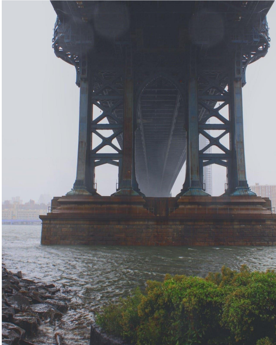
Fig. 2. Manhattan Bridge, October 2018. Down under the Manhattan Bridge on the Brooklyn side there are numerous footpaths and tidal Marshes along a path named John Street. During a driving nor'easter, I left the safety of the path and faced the tower. The conditions provided density that complements the magnificence of this 1901 structure. Photo credit: Denice Martone.
