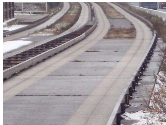
Figure 6 A Close Look at Guiderail
