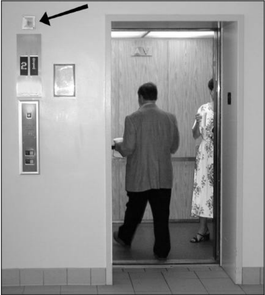
Figure 2.2 Transmitter Cover and Placement
