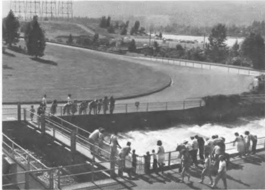
The fish ladders are a significant tourist attraction.
