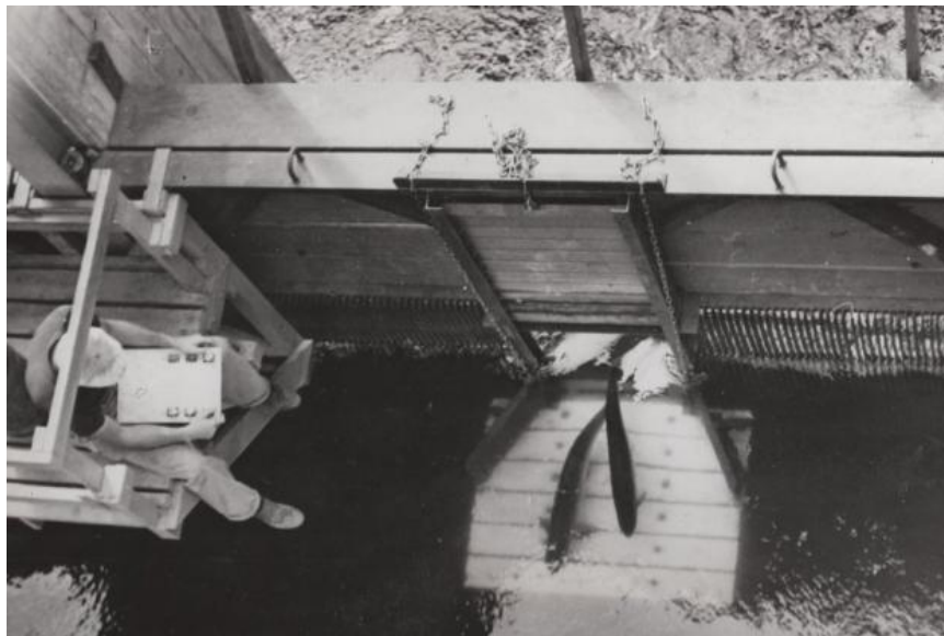
Figure 36 A “fish counter” sits on wooden platform (left) documenting fish seen from above as they swim through the dam’s fish gate (center). 317
