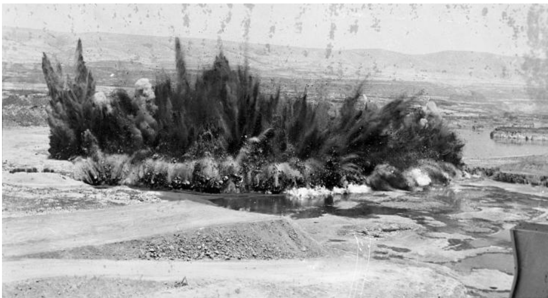
Figure 19 “Final major blast at the Dalles dam, removed 60,000 cubic yards of basalt, more than 20 tons of powder used.” 1956.
