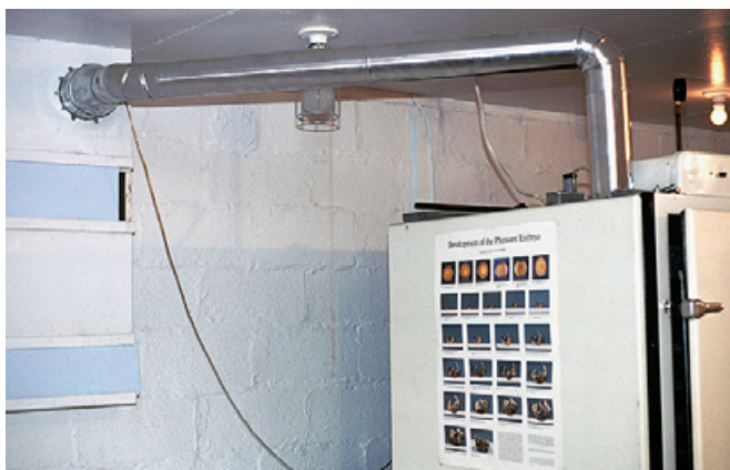
Figure 3. Game bird incubator with an exhaust duct to the exterior of the hatchery.
