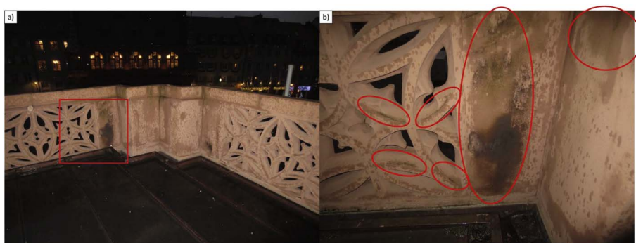
Fig. 11. The Renaissance-Vorhalle during a rain-event (a) and a close-up view of a Mn-rich crust (b). Black crusts and biogenic material develop at surfaces which get wet and remain wet in spite of the hydrophobic silicon resin paint. One can presume that the paint is too thin on these surfaces, or that fissures or cracks allow water to intrude between the paint and the rock. (For interpretation of the references to colour in this figure legend, the reader is referred to the web version of this article.)
