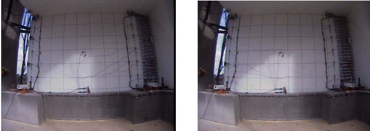
Fig. 8 Extent of flexure-shear cracking at the first story (plastic-hinge region) of the web wall during EQ4 (at instants of time near maximum base rotation)
