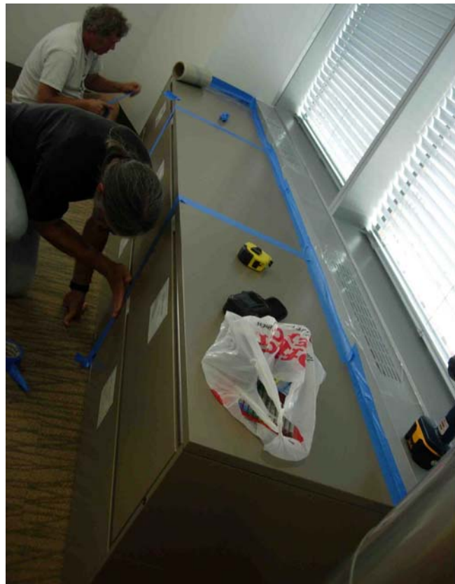
Figure 14: Taping cracks and cabinets at perimeter
