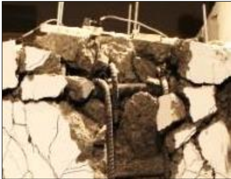
Figure 2.7.8. Apparent opening of the cap tie on top face of Beam 2 as observed upon completion of Beam 2 test.
