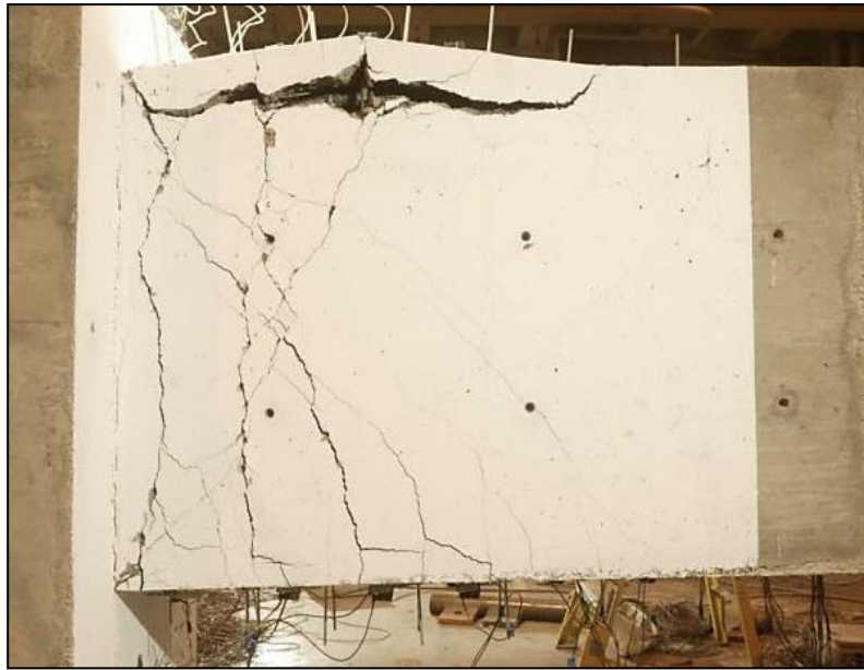
Figure 2.7.2. Beam 1 crack patterns and buckling of the top longitudinal bars (first cycle with peak \theta = -0.027 ).
