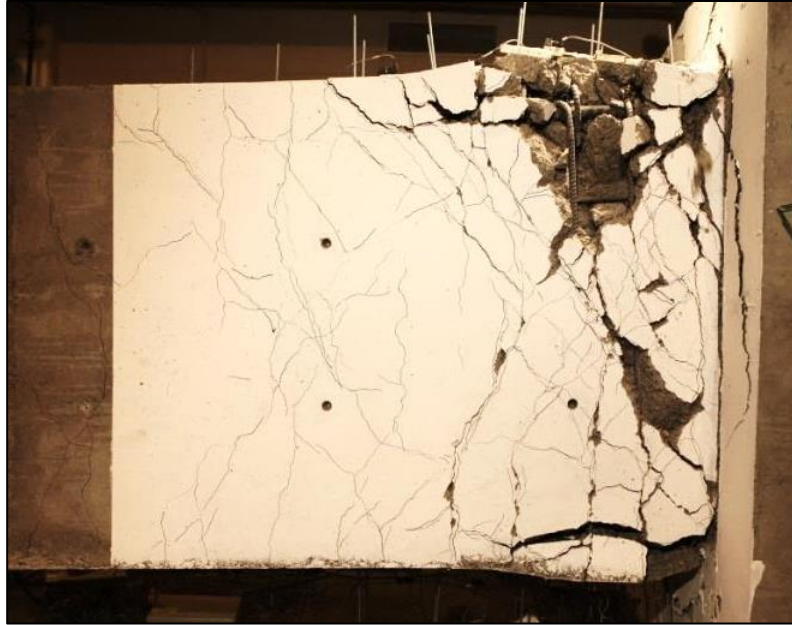
Figure 2.7.7. Buckling of bottom longitudinal bars in Beam 2 ( \theta = 0.053 ).
