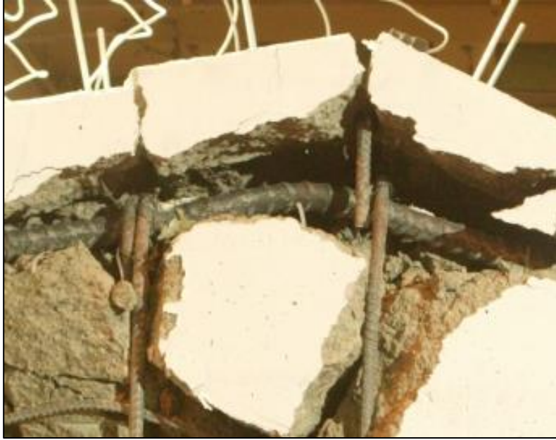
Figure 2.7.4. Stirrup hook opening at the end of Beam 1 test.
