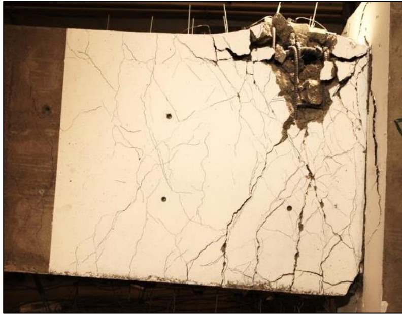
Figure 2.7.6. Crack patterns and buckling of the top longitudinal bars in Beam 2 (first cycle with peak \theta = -0.039 ).
