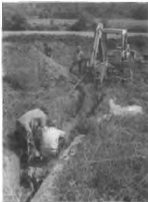
Figure 2.15. Trenching with a backhoe in northern Solvieux Centre
