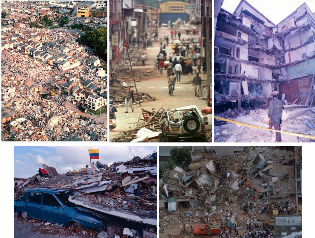
Figure 1.2 Damage observed after the Mw 6.1 1991 Armenia Earthquake. Adapted from El Tiempo (2019).
