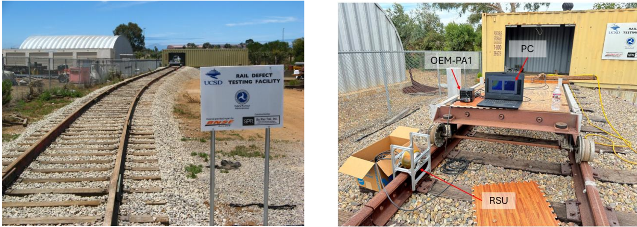
Figure 3.19: Field test at UCSD’s Rail Defect Farm.
