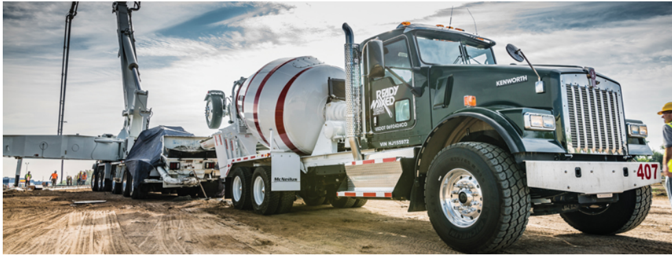
Figure 1: Concrete Mixer Truck in Use
