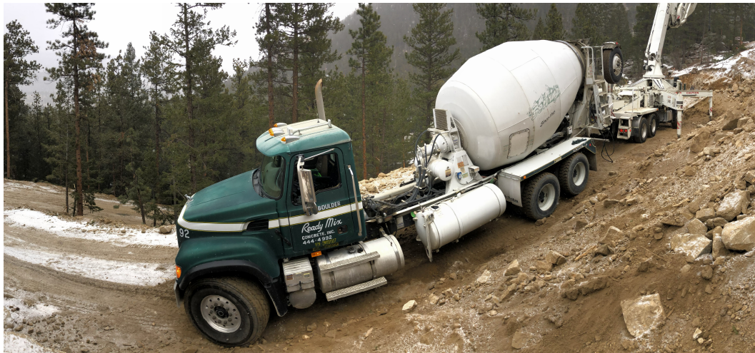
Figure 7: Concrete Mixer with Driver-Side Mounted Water Tank
