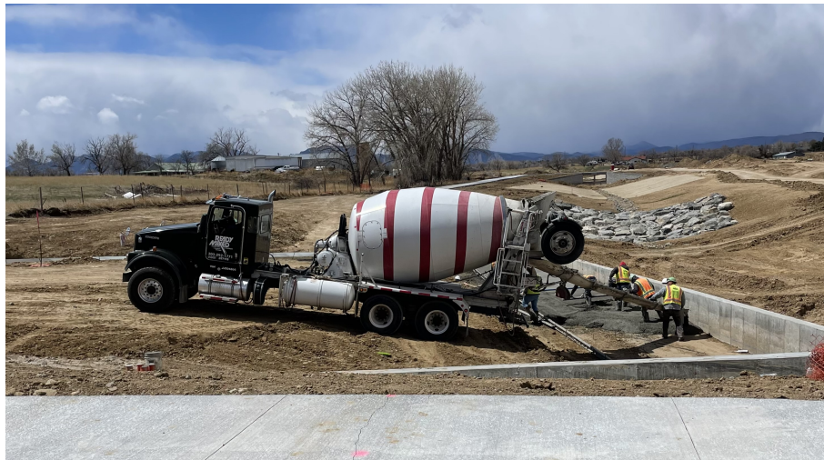
Figure 2: Mixer Truck Pouring Bike Path
